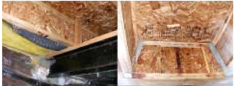
I-Joists and Steel Beam
